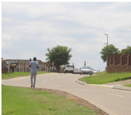
THE COMPLETED MTHAMBAMA ROAD.
