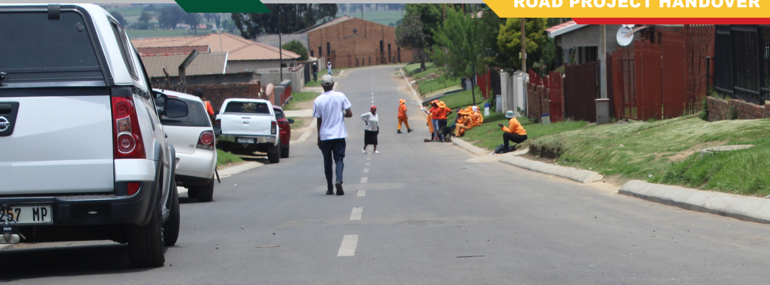
COMPLETED ROAD OF AVENUE STREET.
